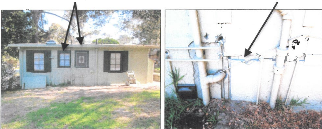
Figures 3 and 4. Left image shows the right side elevation with newer window inserts (arrows). Right image details the right side elevation and shows the Beaverboard siding, overcoated with a stucco finish and covering the original vertical board siding.
